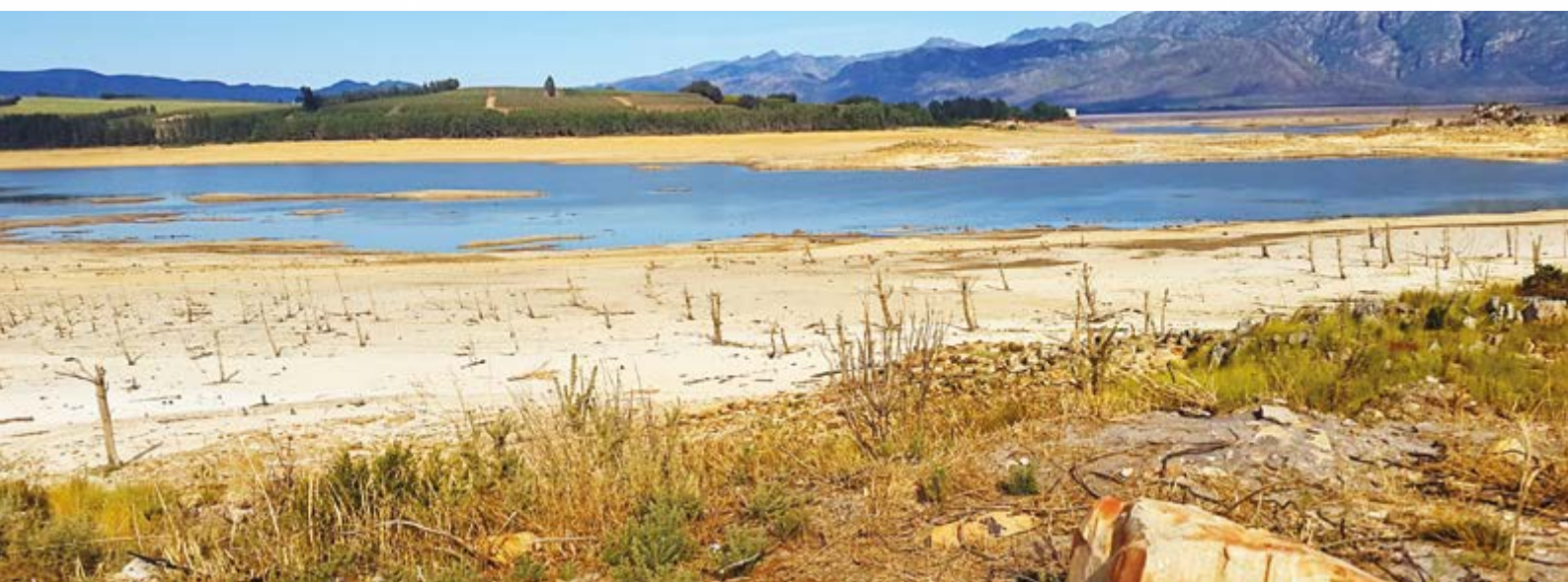
Theewaterskloof Dam outside Cape Town
